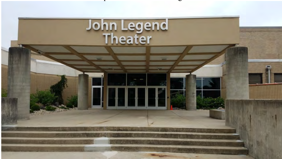
JLT Entrance (Ramp from Parking Lot to the right)
